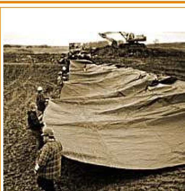
Pulling out a Fabricated Geomembrane Panel
